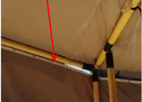
use 25m length 8# khaki rope to pass through the reserved hole
